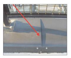
2. Clear scupper area to encourage drainage of rainwater and snow melt. Scuppers located under decking are covered with a pigeon-deterrent metal screen—deck boards will have to be removed to clear any debris that collects inside the screen.
