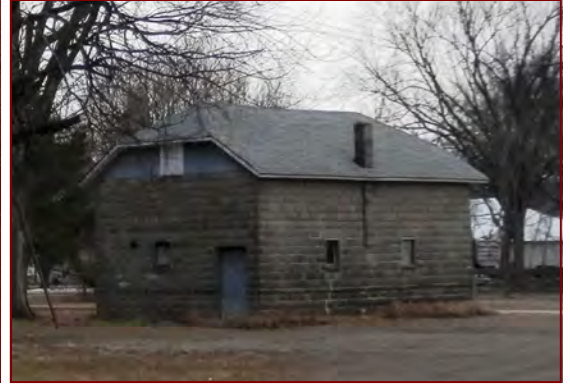
NE CORNER OF HISTORIC BLOCK BLDNG
